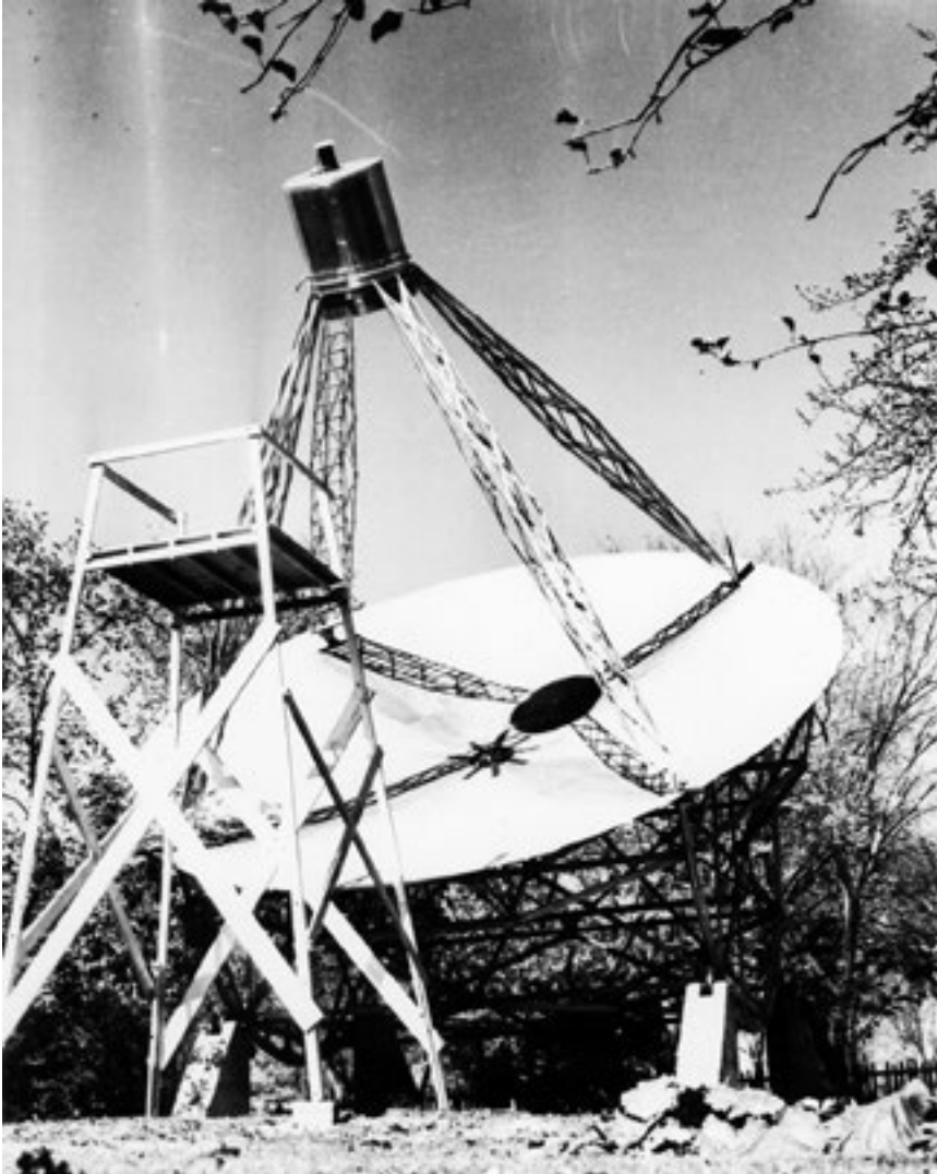
Image 4. First radio telescope built by Grote Reber in 1937. Credit: NRAO-Green Bank.
